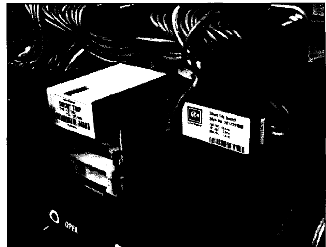
Figure 3-36 Shunt Trip Switch Installed
