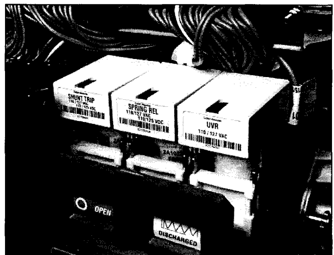
Figure 3-39 Shunt Trip, Spring Release and Undervoltage Release Installed
