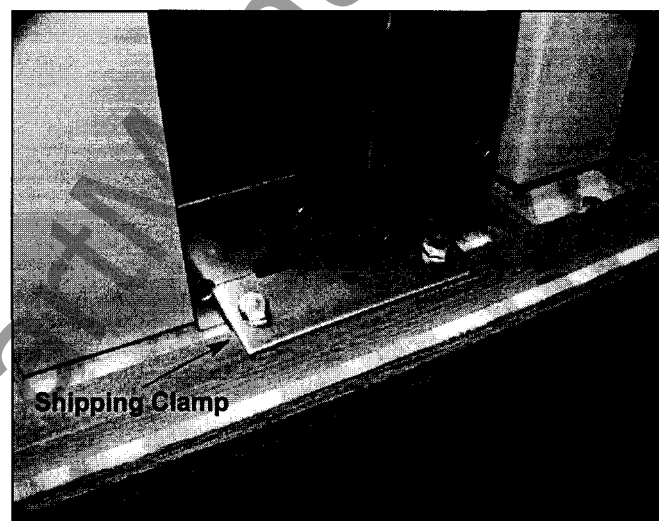
Figure 2-1 Shipping Clamps for Drawout Circuit Breaker
