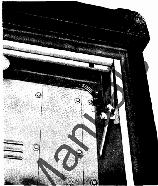
Fig. 14 Tandem Lock For Outdoor 13.8 Units
