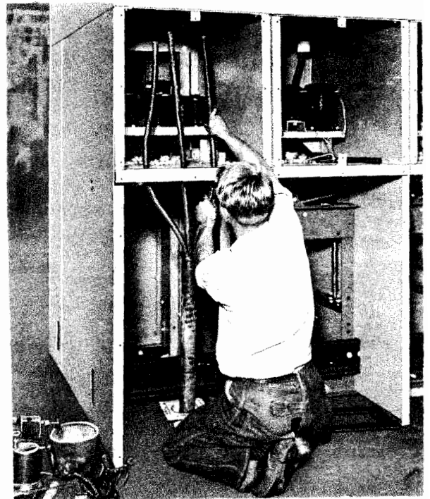
Fig. 25 Approximating Final Position
