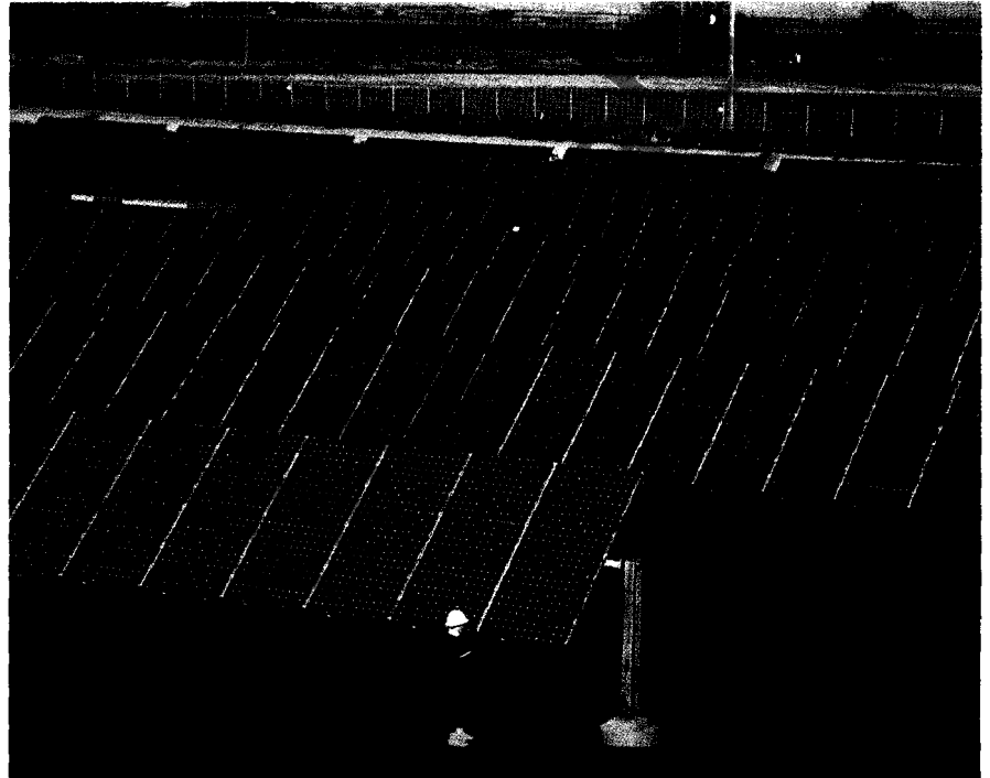
High Efficiency Photovoltaic Solar Electric Array
