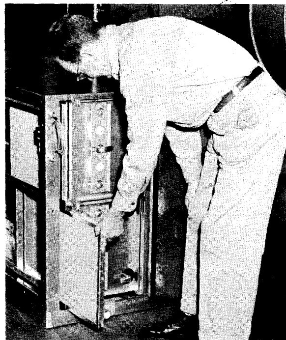
Figure 17. Installing After-Filters
