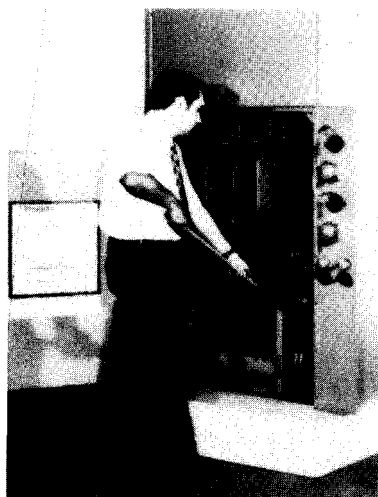
12 Push contactor onto load stabs.
