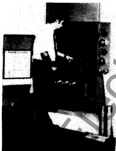
15 Replace the three power fuses. Follow FUSE INSERTION instructions shown on the starter door.
