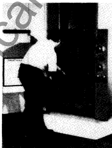
16 Rotate blowout irons forward and down. CAUTION! Make sure the 3 arc boxes and 4 phase barrier are in place. Door will not close if blowout irons are in the wrong position. Close and latch the starter doors.
